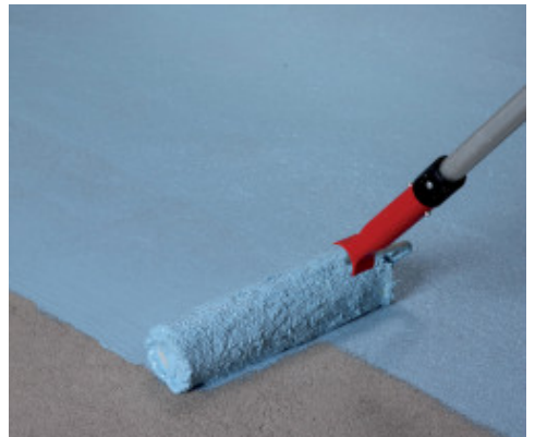
Application of the first coat of Mapelastick AquaDefense on a screed
