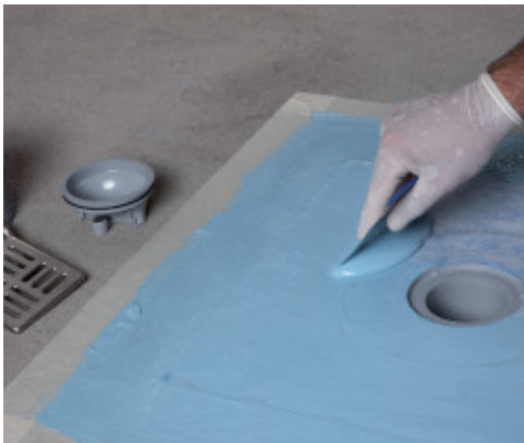
Impregnating Drain Vertical fabric with Mapelastick AquaDefense
