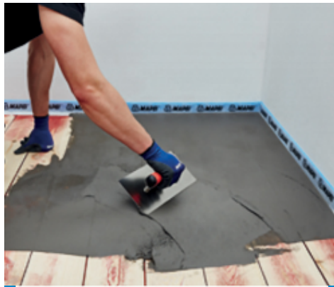
Application of Planipatch Xtra + Latex Plus on wooden substrate
