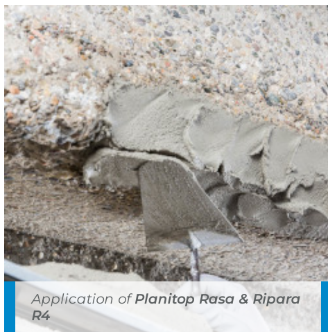
Floating of Planitop Rasa & Ripara R4
